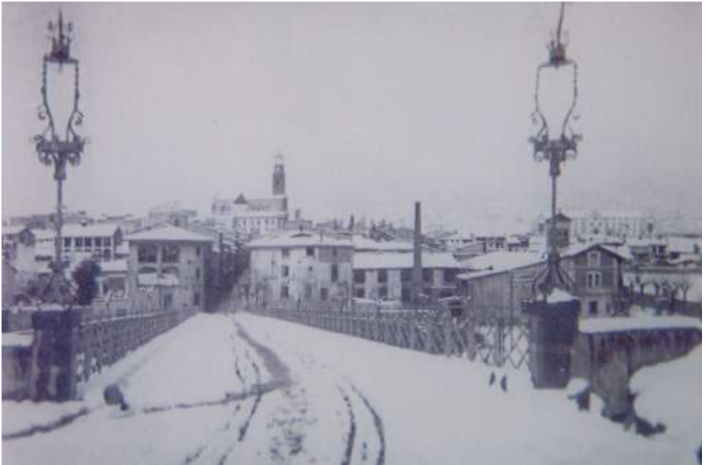
Can Dordal (al frente, a la izquierda), la casa familiar de Juan Dordal Pujadas, se encontraba en un extremo del puente de Can Moles, en Manlleu. Can Dordal (opposite, on the left), Juan Dordal Pujadas' family home. It was at one of both ends of the Can Moles bridge, in Manlleu.
